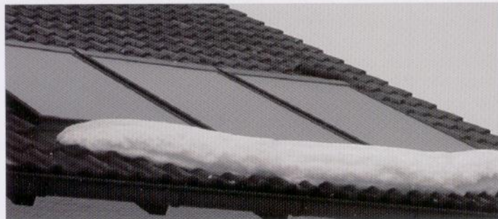
pictured above: snow that has slid down the surface of a solar flat plate collector photos courtesy of Center of Excellence For Solar Engineering at Ingolstadt University
